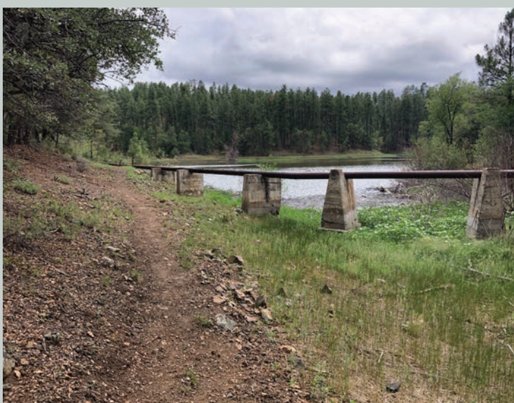
Old water line that took water into town
