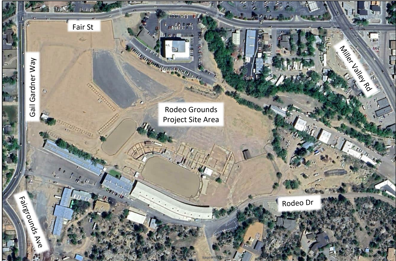
Figure 2 – Existing Site Condition (May 2023):
