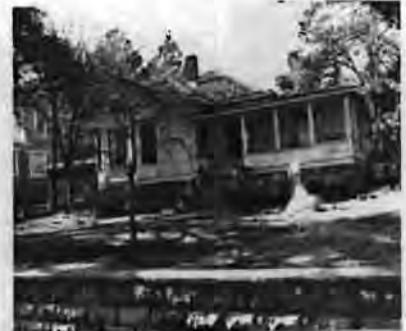
Walter Hill House, 138 Park Avenue (c. 1910); Elements of Bungalow and Queen Anne Styles, Bellcast Hip Roof with Projecting Front Gable, Leaded Glass, Classical Columns, Large Stone Retaining Wall
