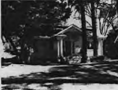
Bungalow, 716 Country Club Drive (1926); Irregular Plan with Symmetrical Massing, Centrally Located Porch with Arched Ceiling and Skirted Returns in Deep Frieze Boards Supported by Classical Columns
