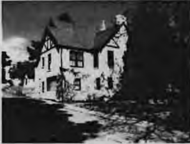
Tudor Revival, 336 Park Avenue (1933); Steep Gables, Stucco with Half-Timbering at Gables, Tall Windows with 9/1 Pane Design, Terraced Stone Wall at Front of Property
