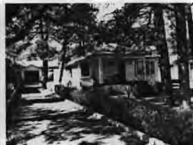
Albert Bork House, 222 Park Avenue (c. 1910); Bungalow, Wood Shingle Siding, Diamond-Patterned Upper Window Panes, Windows Banded in Threes, Stone Fireplace
