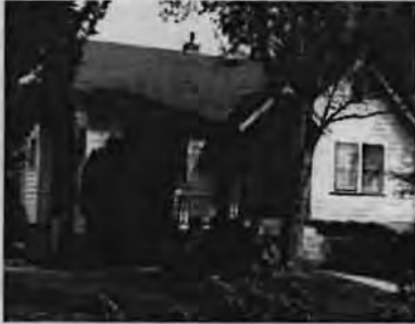
Revival Style Elements, 417 Perry Street (c. 1935); Side Gable with Off-Set End Gable Projecting to Street, Small End Gable Over Porch on Brick Columns, Brick Chimneys, Paired 9/1 Wood Windows
