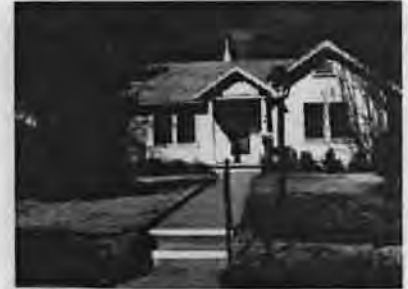
Bungalow and Revival Elements, 370 Park Avenue (c. 1931); Asymmetrical Massing with Central Entry, Louvered Vents and Exposed Beams Project Beyond the Fascia, Classical Columns Support Small End Gable at Entry
