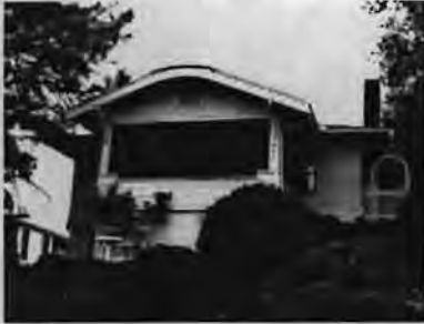
Bungalow, 541 Hill Avenue (c. 1920); Wood Siding Flares at Top of Basement Wall, Arched Gable Supported by Truncated Columns at Porch, Decorative Brackets Support Exposed Beams, Native Rock Outcroppings Remain at Front
