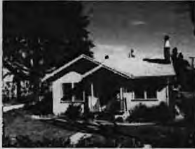
Bungalow, 616 Country Club Drive (c. 1928); Side Gable Roof with Off-Set Gable at West End, Lesser End Gable at Porch, Decorative Beams, Classical Columns, Paired 4/1 Wood Windows
