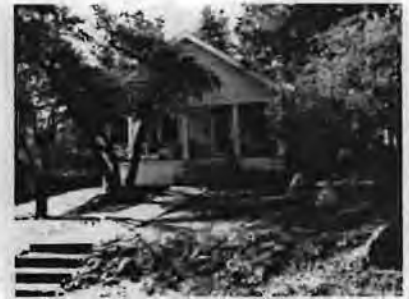
Bungalow, 626 Glendale Avenue (c. 1930); Large Front Veranda Under End Gable Supported on Truncated Wood Columns, Clapboard Siding. Simple 1/1 and 2/1 Wood Windows
