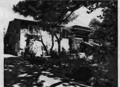
Bungalow, 222 Vista Drive (c. 1926); Rectangular Plan, Shallow Side Gable with Central Shed Dormer, Prominent Entry Stairs with Stone Sidewalls, Shiplap Siding, Multi-Pane Windows Flanked by 1/1 Double-Hungs, Exposed Rafter Tails, Native Landscaping and Rock Walls
