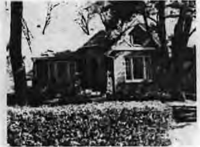
Tudor Revival, 712 Country Club Drive (1928); Brick with Half-Timbered End Gable, Stuccoed Hexagonal Tower at Entry, Stone Wall at Porch, 10-Lite Windows Flank 8/1 Windows at Front
