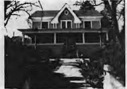
Amy Hill House, 144 Park Avenue (1906); Elements of Queen Anne and Revival Styles, Central End Gables with Central Side Gable at Entry, Wide Fascias, 1/1 Wood Windows with Wide Trim, Classical Columns at Front Porch
