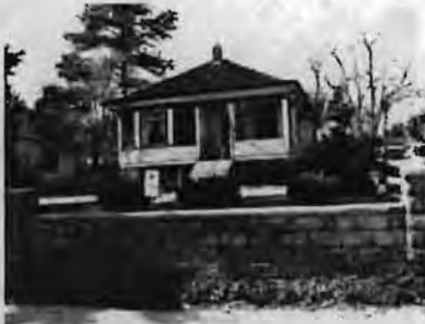
Samuel E. Wallace House, 132 Park Avenue (1908); Simplified Bungalow, Bellcast Hip Roof, Soffited Eaves with Wide Frieze, Bay Window, Re-entrant Porch
