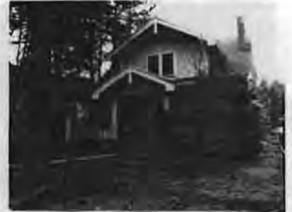
Bungalow & Prairie School Styles, 338 Park Avenue (c. 1931); Central Entry Under Large Gabled Dormer, Wide Fascias, Decorative Brackets Under Exposed Beams, Jigsawed Balustrades
